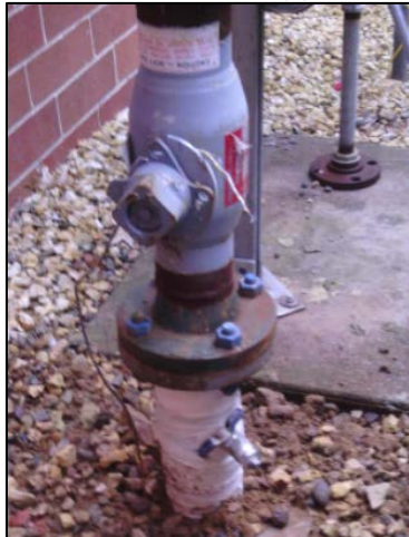
9) Lee Lohman Arena, Saint Ambrose University, West Lombard Street MidAmerican rewrapped the riser.
