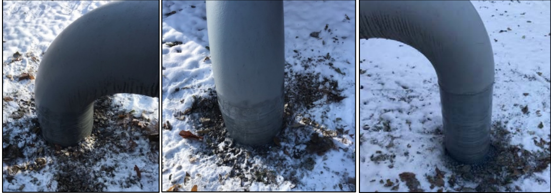
6) Multiple Risers, QCIA16 Blackhawk TBS MidAmerican rewrapped the risers.
