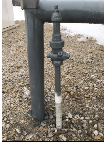
4) DRS #122 at Locust Street MidAmerican rewrapped the riser.
